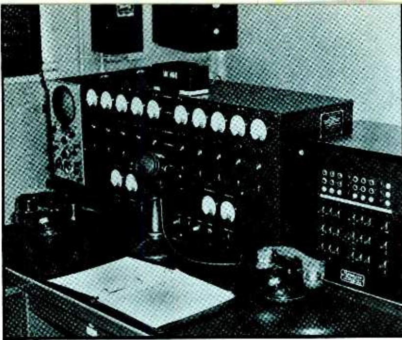
Central control room of fireboat system. Telephone monitor board, receiver, frequency monitor and power supply unit
